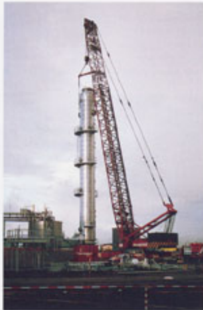
Dordrecht — A 140 tonne furnace with accessories was transported for a major extension of a Dupont petrochemical plant in Dordrecht. Somewhere else on the site a 90 tonne reactor column was erected and positioned.
